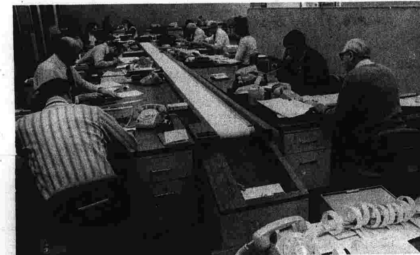
The Herald uses a conveyor system to move news copy from the reporters to desk men for final editing. The editorial department, as well as the other departments, are equipped with Olivetti OCR typewriters. OCR is short for Optical Character Recognition. On the typewriter, the reporter actually codes his story, or instructs the all-electronic type-setting equipment as to the size and style of the type desired.
